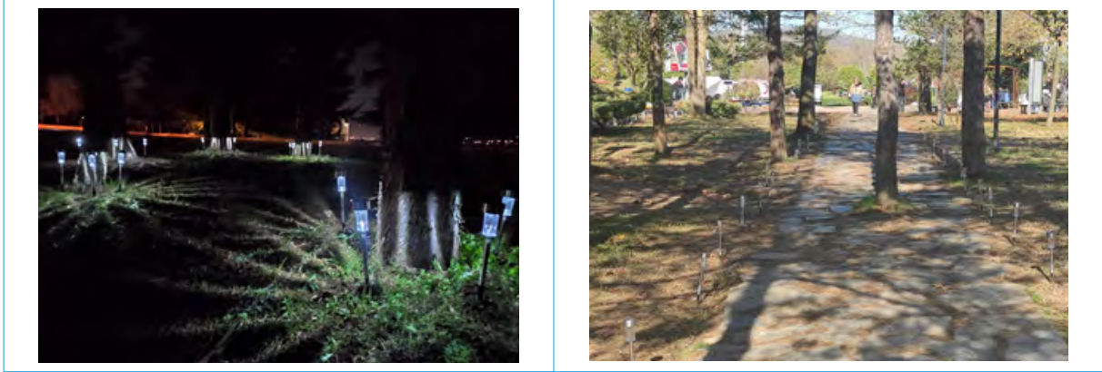
Figure 30: Lighting Solar panel lighting around campus
