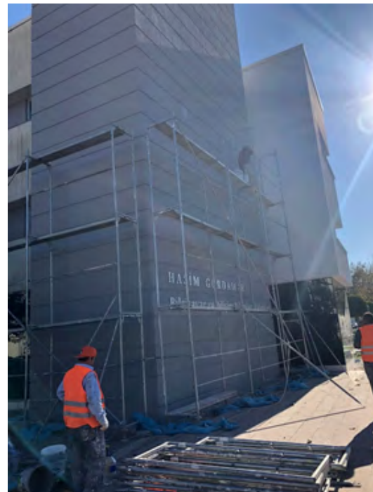
Insulation application on building exteriors
