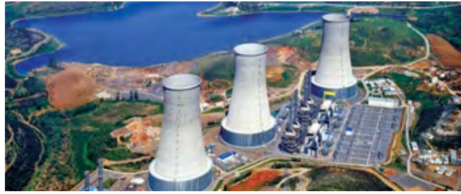
2. Electricity generation plant from natural gas combined cycle in Sakarya
