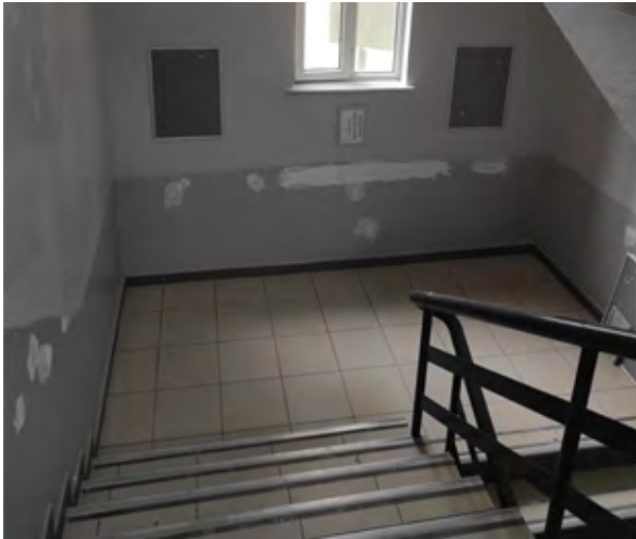
Internal maintenance and repair work of building
