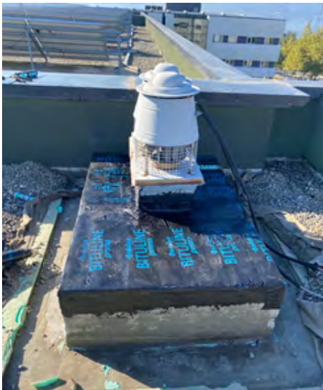
Maintenance and insulation process of air conditioning system in the building
