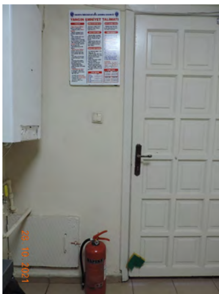
2. Standard Room with fire instructions and precautions
