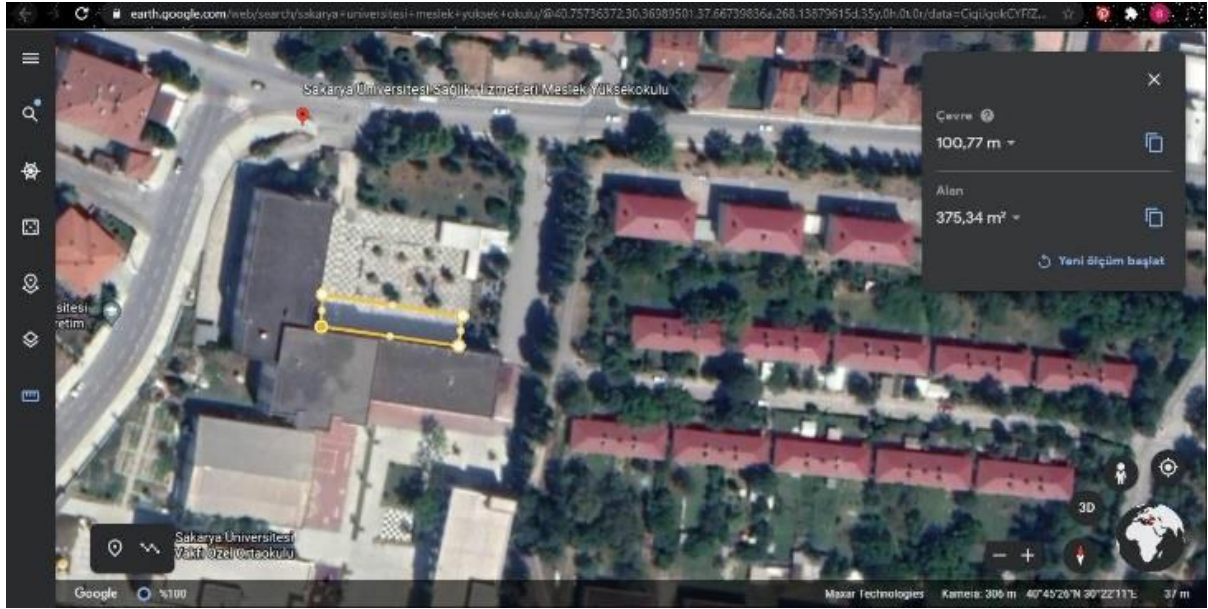
Figure 48: Parking Area - Health Services Campus
