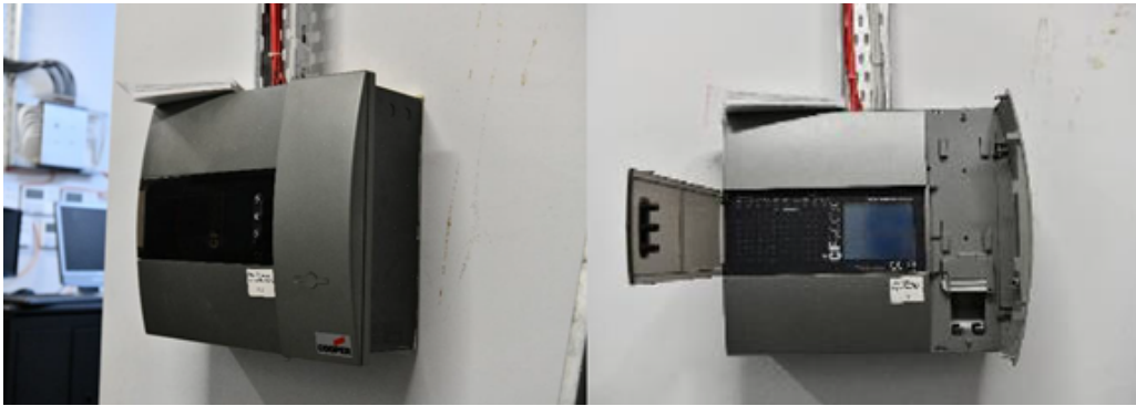
Fire Alarm Control Center
